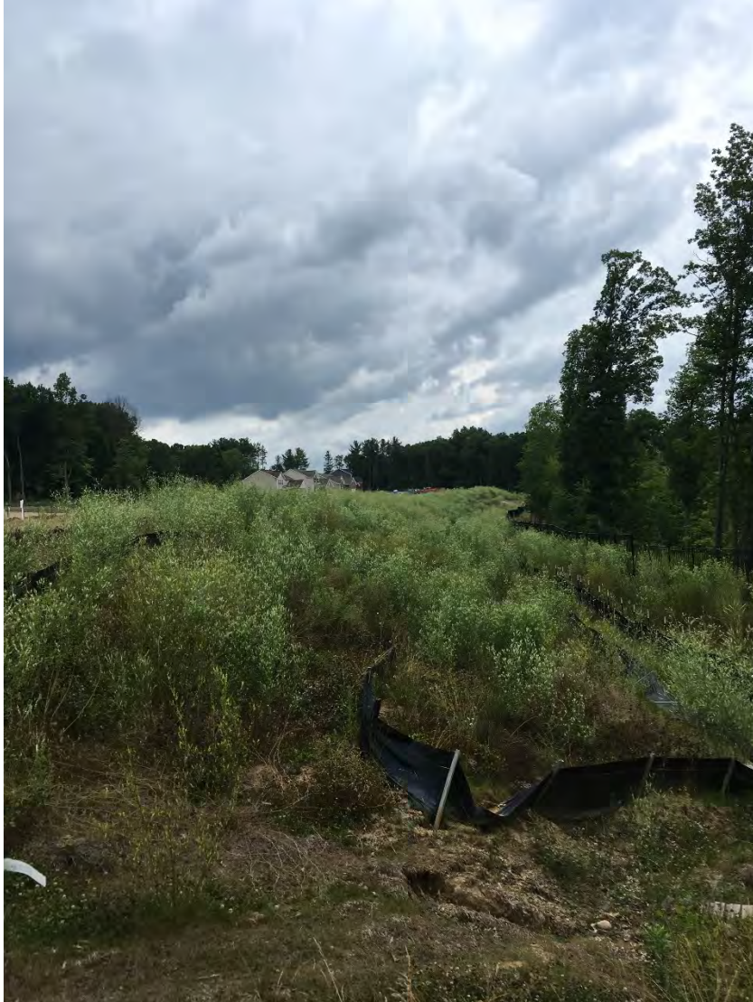
Non maintained silt fence found. Photo taken 7/10/19
