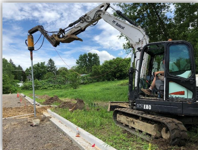
Fig.3 / Helical Pier Installation(Vertical)
