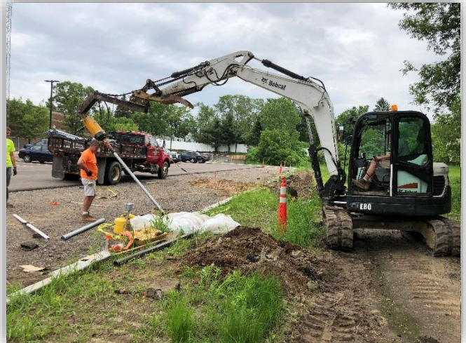
Fig.2 / Helical Pier Installation(Inclined)
