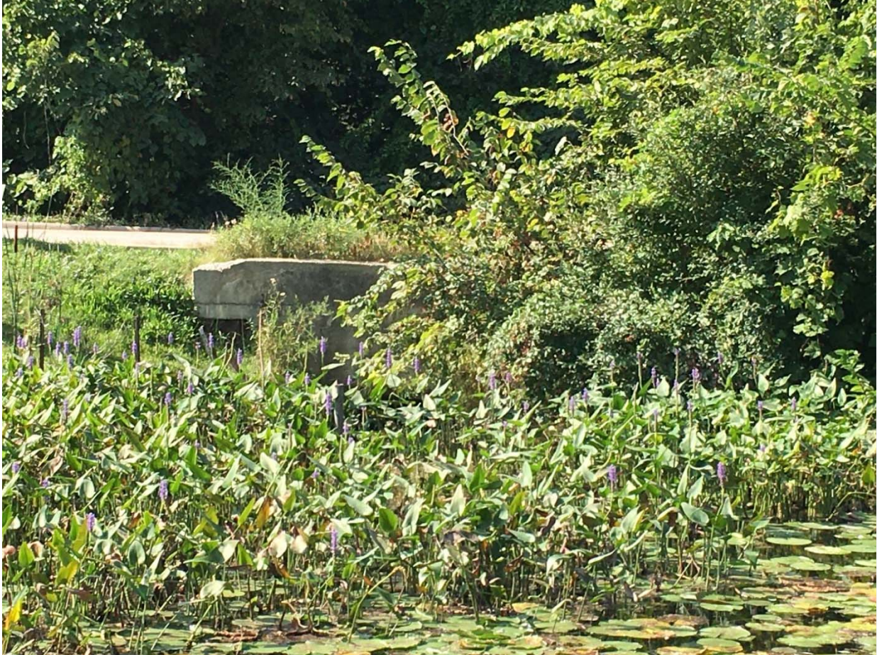
LOOKING SOUTH TOWARDS BLAINE ROAD – UPSTREAM CONCRETE HEADWALL IN BACKGROUND
