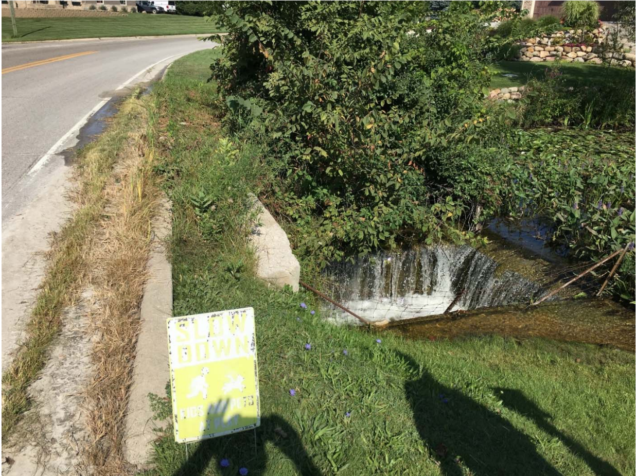
LOOKING WEST AT OVERFLOW STRUCTURE
