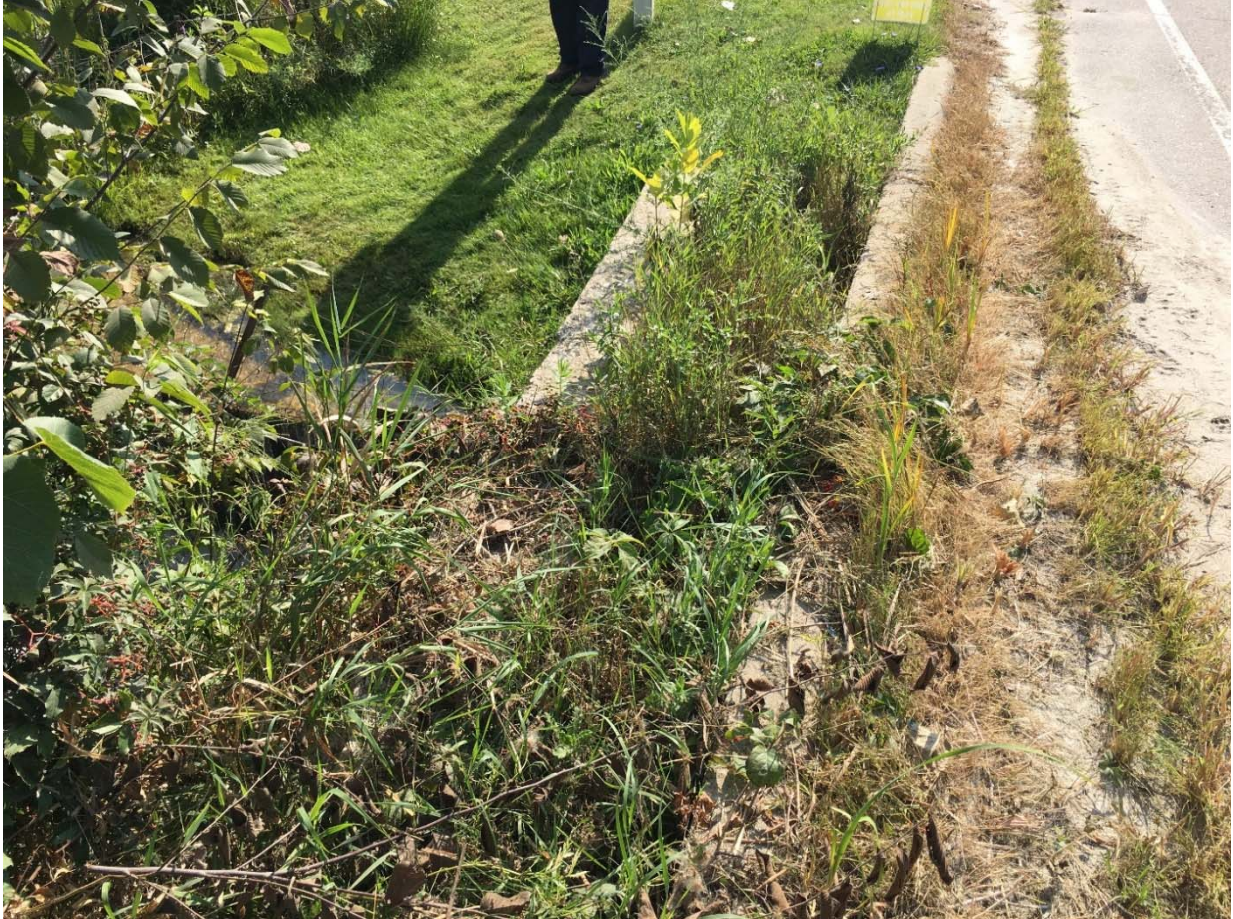
LOOKING EAST AT CONCRETE HEADWALL
