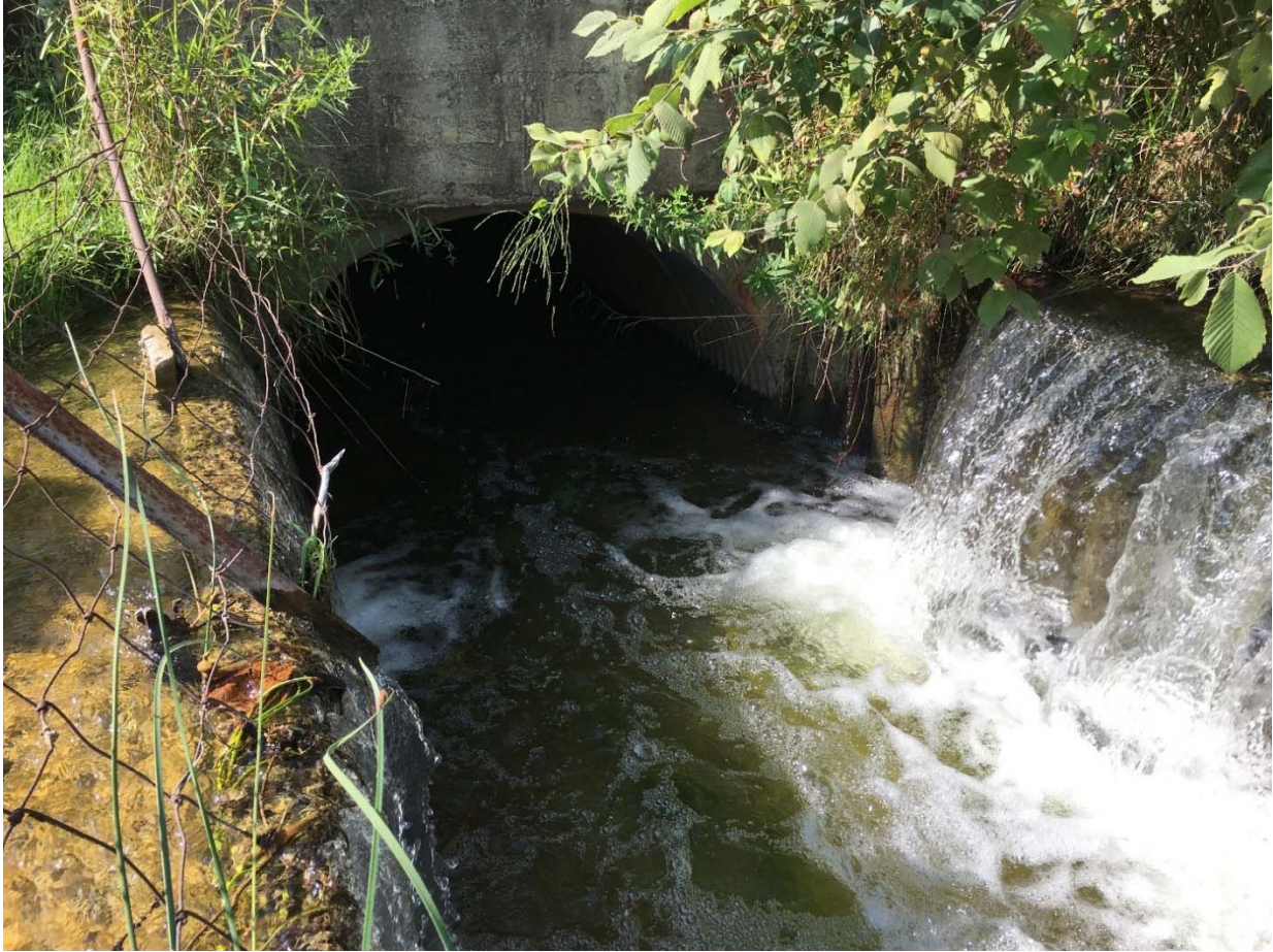
LOOKING SOUTH AT OVERFLOW STRUCTURE WITH OUTLET PIPE AND CONCRETE HEADWALL
