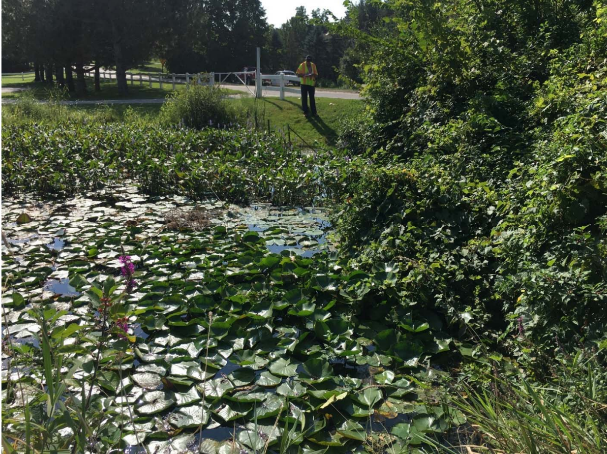
VIEW OF UPSTREAM CHANNEL SHOWING HEAVY WATER VEGETATION GROWTH
