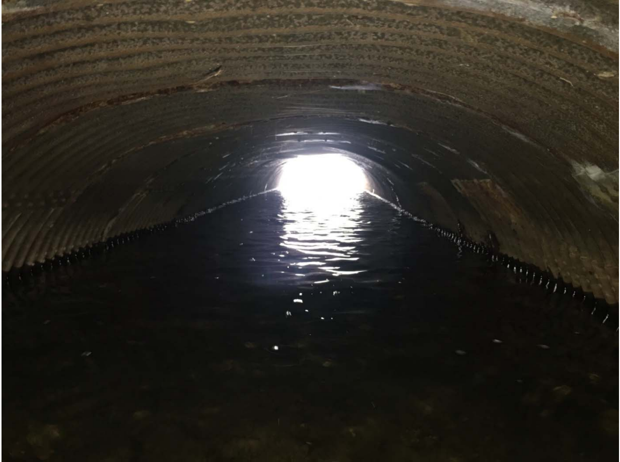
VIEW INSIDE OUTLET CMP PIPE LOOKING UPSTREAM
