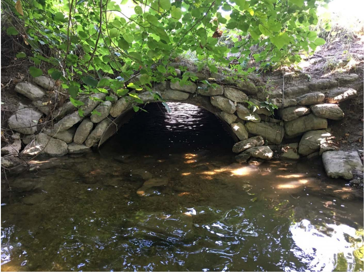
VIEW OF DOWNSREAM OUTLET CMP PIPE
