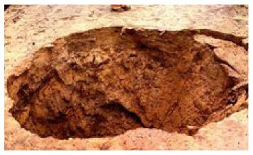
Above: Sinkhole on the crest of an earth dam. The reservoir was lowered and a cavity was found under the sinkhole.
