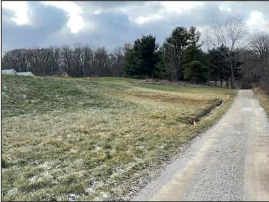
Image 4: Looking west along the driveway at the toe of the embankment. The seepage area is visible to the left of the driveway (photo date: 12/7/2021).
