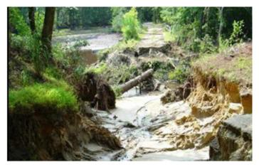
Above: Seepage that developed where the root ball of a tree pulled out of the ground near the downstream toe of the dam.
