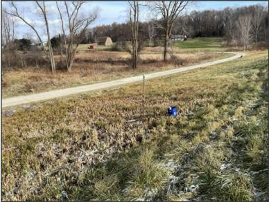
Image 5: Looking northeast at the seepage area. The blue bucket is located near the upstream edge of the seepage (photo date: 12/7/2021).
