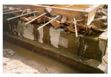
Weep holes with screens to control seepage.
