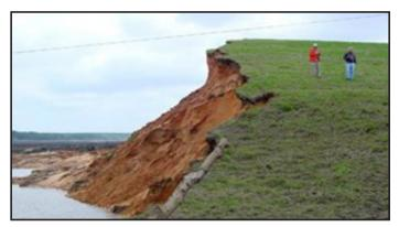
Failure at a dam caused by internal erosion of the soil abutment.
