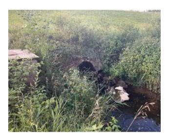
DESCRIPTION: Looking upstream at headwall failure
