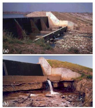
(a) A spillway outlet area as originally constructed.(b) Severe erosion has undermined the spillway outlet and threatens the overall structural safety of the spillways.
