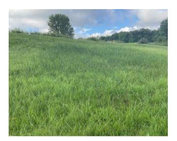
DESCRIPTION: Looking west at saturated ground on downstream slope of embankment
