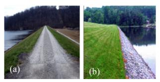
(a) Crest with a good cover that will reduce the effects of vehicular traffic.(b) This slope is well maintained with rock riprap along the shoreline.
