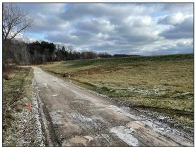
Image 3: Looking east along the driveway at the toe of the embankment. The seepage area is visible to the right of the driveway in the background of the pink stake (photo date: 12/7/2021).
