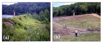
(a) Embankments covered with trees and brush makes inspections difficult. (b) Cleared of trees and brush, this embankment is much easier to inspect, but needs a good vegetal cover.
