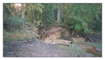
Tree roots growing into the dam's earth embankment causing failure.
