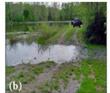
*(a) Embankment crests with vehicle ruts will collect water and weaken the embankment. (b) Crest beginning to overtop in low area. This could lead to erosion and failure of the dam.*
