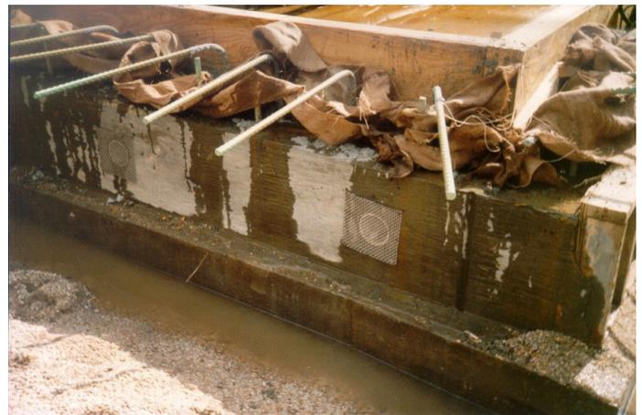
*Weep holes with screens to control seepage.*
