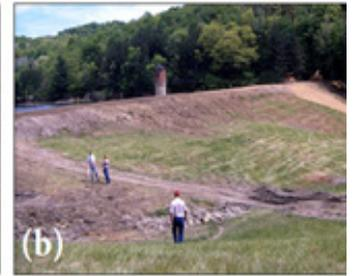
*(a) Embankments covered with trees and brush makes inspections difficult. (b) Cleared of trees and brush, this embankment is much easier to inspect, but needs a good vegetal cover.*
