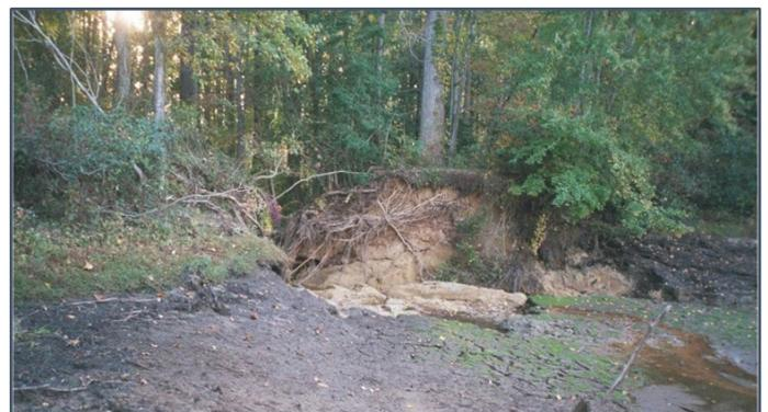
*Tree roots growing into the dam's earth embankment causing failure.*
