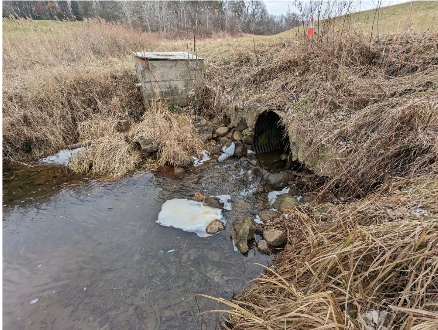
Figure 9a - Dam outlet, measured 40" CMP, corroding inside and deformed, headwall is falling apart and has sinkhole between road and outlet. Box is the irrigation system used for watering the nearby pumpkin patch, no longer in use.
