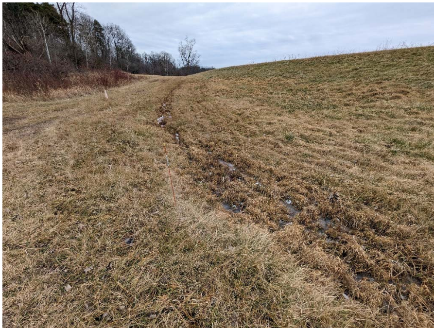
Figure 5a - Looking south uphill at seepage flow.
