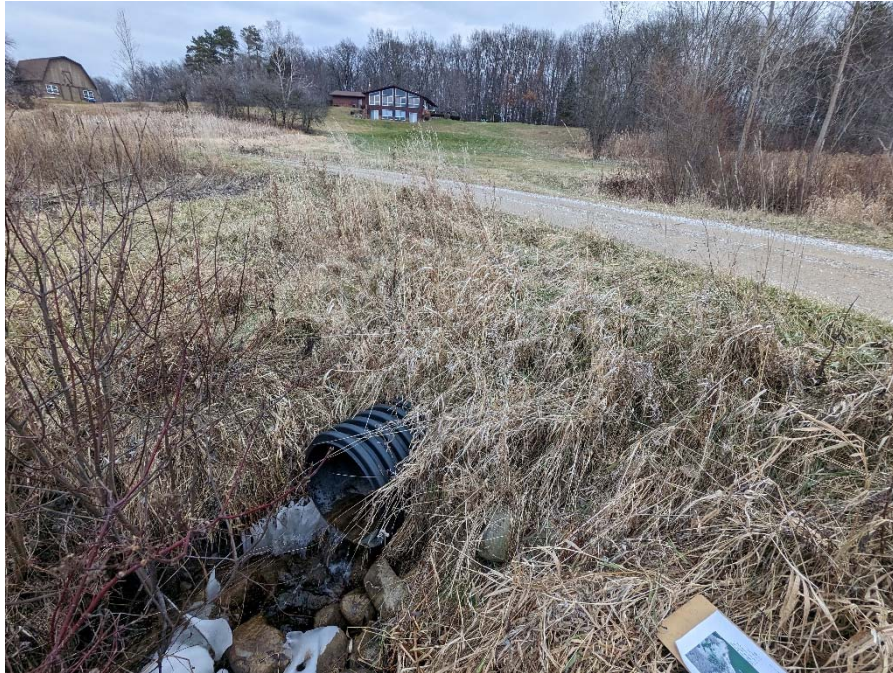
Figure 4 - Looking north at 24" HDPE culvert.
