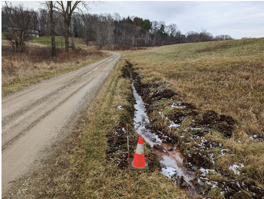
Figure 10 - Looking east at hand dug ditch to collect seepage flow from lake.
